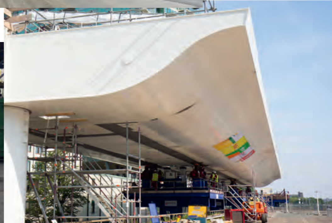
Hammer piece and deck A
