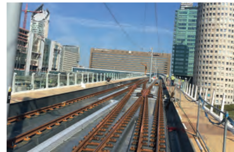
Track with points on the bridge deck
