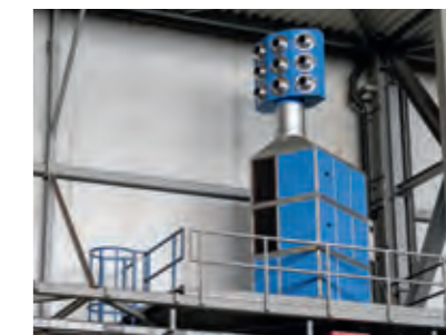
Extraction of welding gas at Smulders Projects in Hoboken
